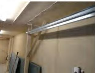
Photo 2: Water trapped behind perfect barrier assembly leaking into the garage below
