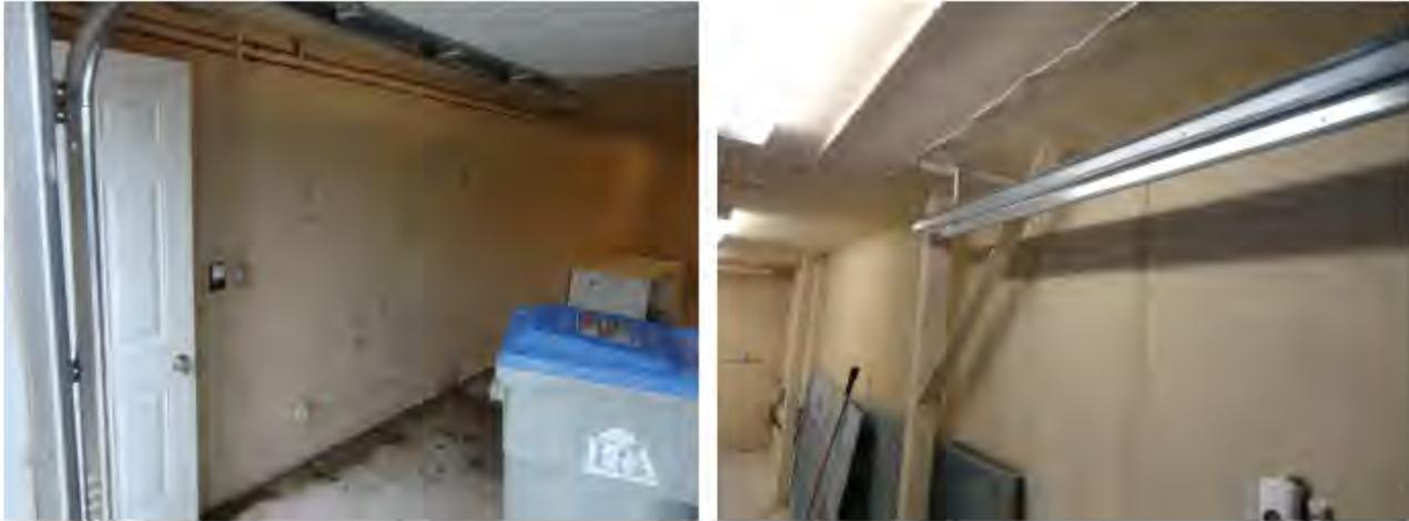
Photo 2: Water trapped behind perfect barrier assembly leaking into the garage below
